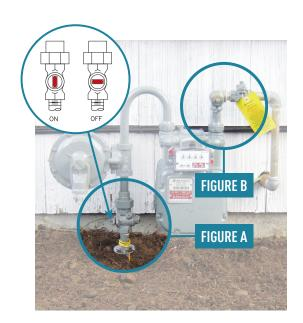
• Turn the valve head crosswise (perpendicular) to the pipe and it will be in the OFF position.
